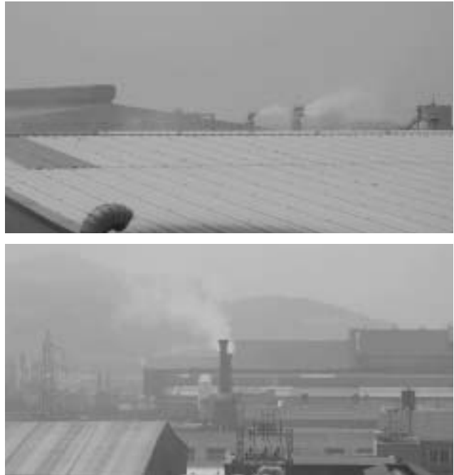
Fig. 3. Photographs of plume emitted from tenter facilities.
